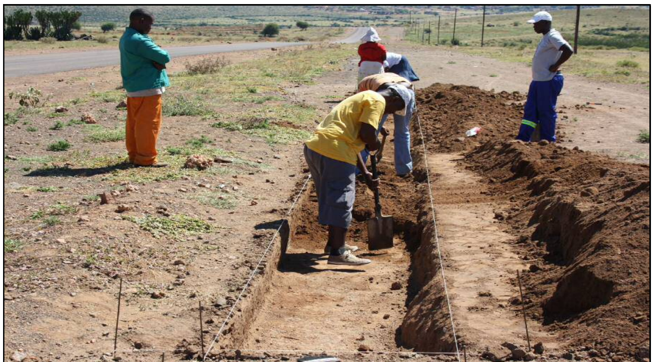
Figure 7: Excavation of the first trench
