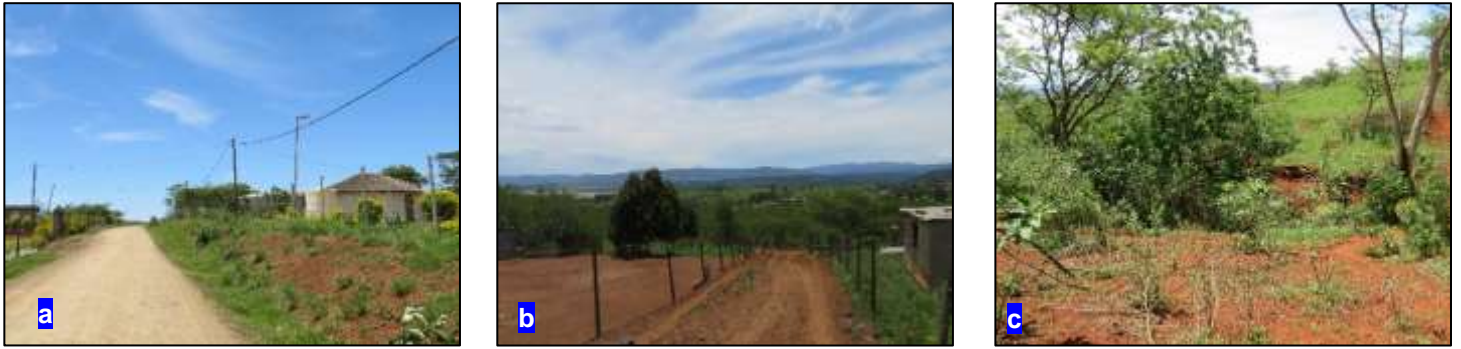
Figure 17: (a) View of an existing formal gravel road within the Thokozani project area where the pipeline will be placed adjacent/within; (b) View of an existing informal gravel road within the Thokozani project area where the pipeline will be placed adjacent; (c) A typical drainage line on site which the pipeline will either be within 32m or cross.
