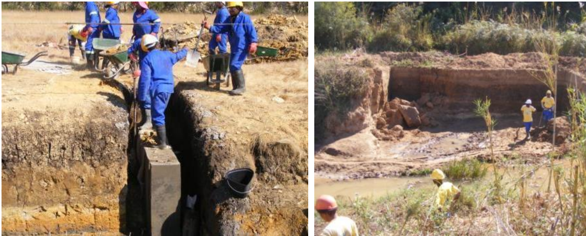
A buttress weir being built and a site being prepared by the Implementing agents
