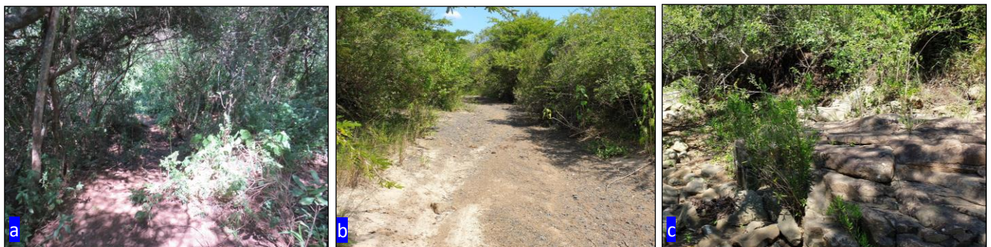
Figure 14: (a): Dense vegetation surrounds a path leading towards WC4; (b): Overview of the Matshitsho river's wide river bed, where the pipeline will cross at WC24 and WC25; (c): Hardrock was noted along portions of the water pipeline.
