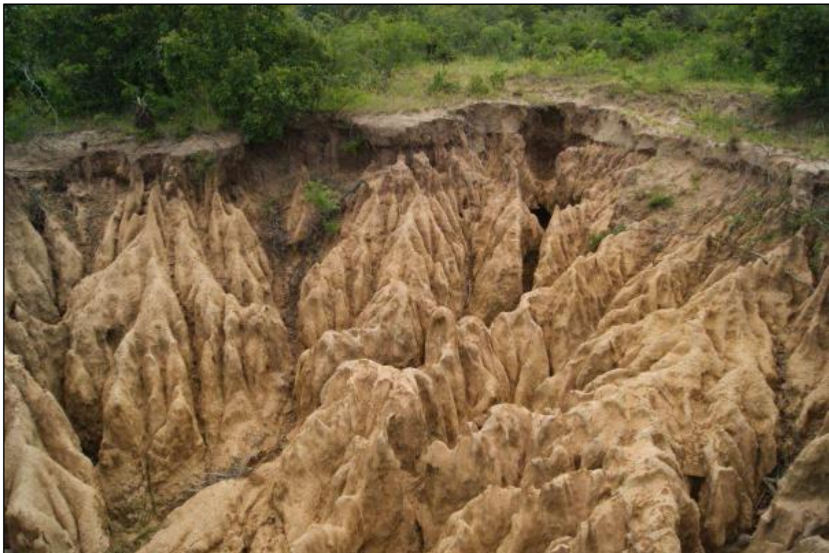
Figure 25: Substantial erosion observed within the watercourse associated with the Msebe project area
