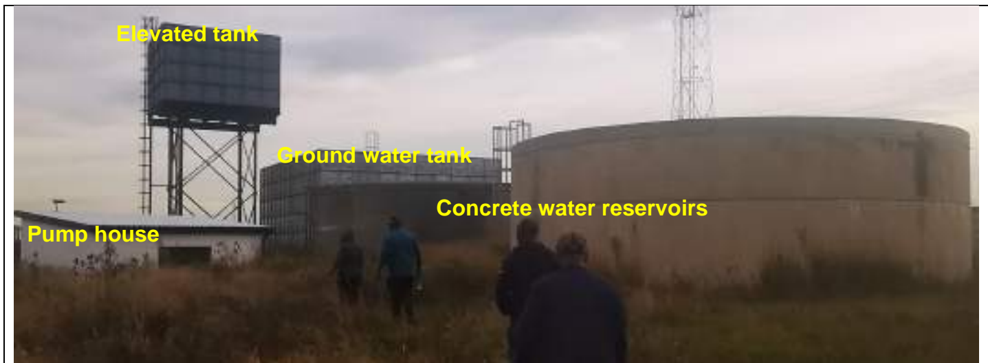
Figure 15 Potable water storages
