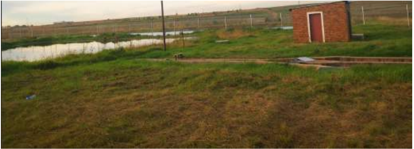
Figure 18 Wastewater Treatment Works
