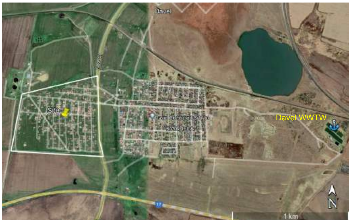
Figure 17 Wastewater Treatment Works
