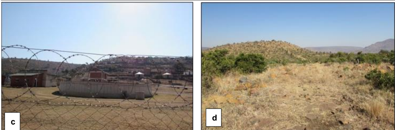
(c) Sampofu WTW water reservoir; (d) Existing servitude that the 200mm pipeline will traverse.
