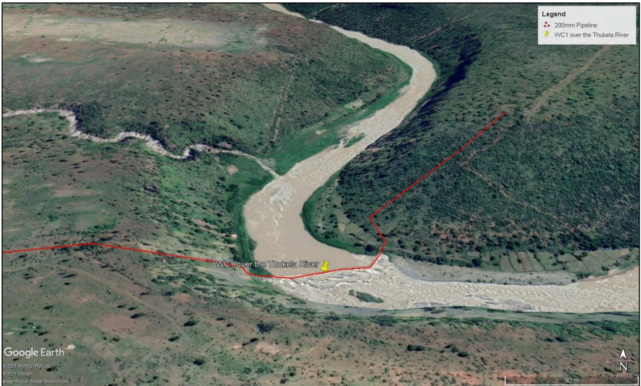
Figure 8: Google Earth Image Showing a Terrain Profile of the 200mm Pipeline over the Thukela River at WC1. Source: Google Earth Pro, 2020.
