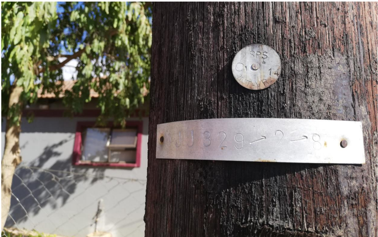
Shows the existing powerline
