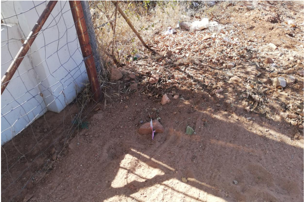
Photo 1: Shows the peg, where the pole will be planted
