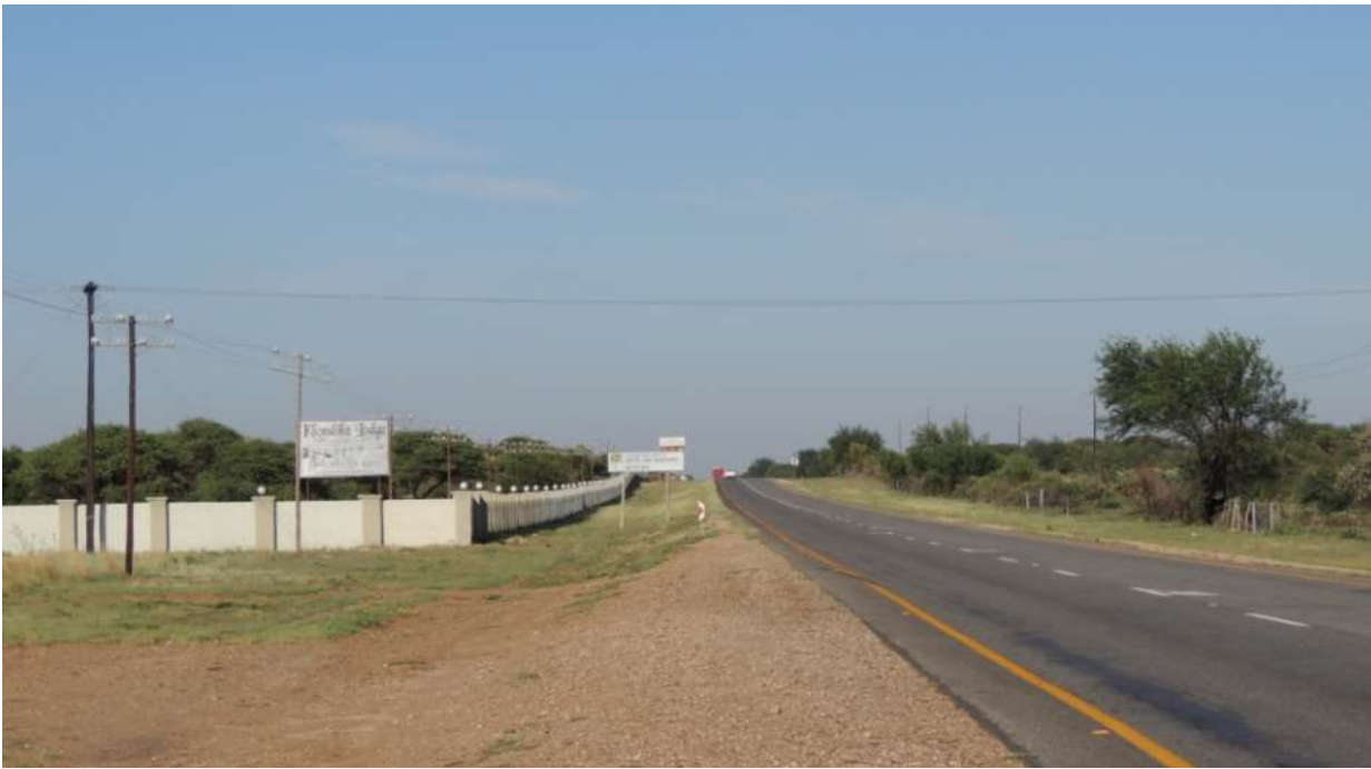
Figure 27: Photograph of the N14 National Road
