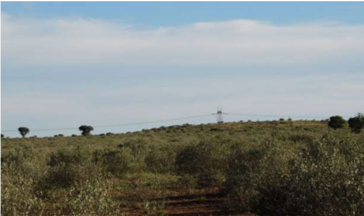
Figure 40: Photograph 6 taken in a southerly direction of the existing Eskom 400kV power line along which the proposed project power line is proposed.
