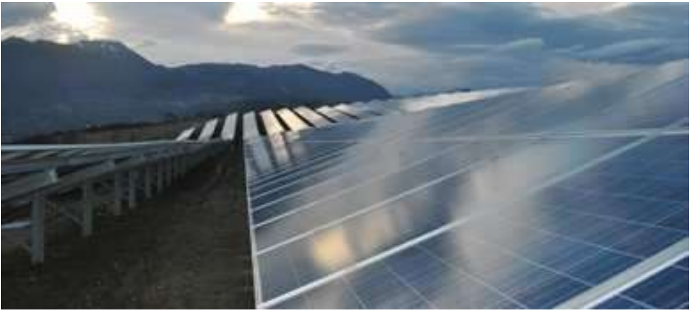
Figure 6: Examples of Fixed Rack Structures
