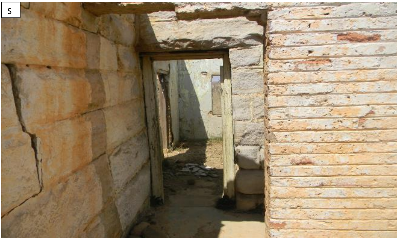
Plate 19: Photo S , showing remaining wooden frames. Note the cracks on the buildings..
