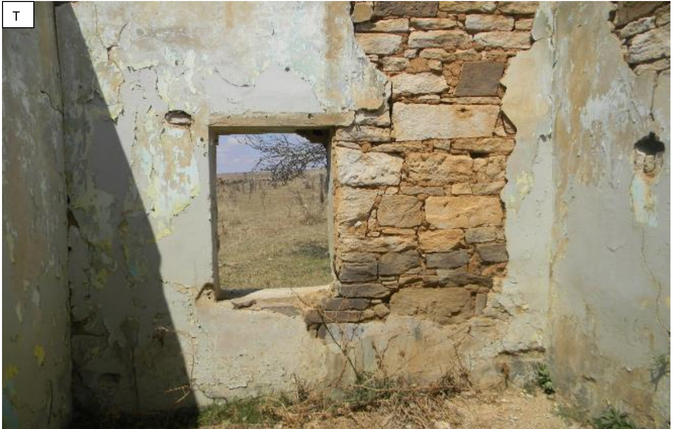
Plate 20: Photo T , showing sections of the building which are collapsing due to abandonment and exposure to harsh weather conditions.
