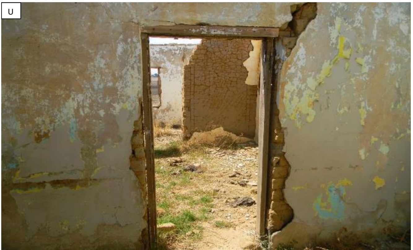
Plate 21: Photo U , showing remaining wooden frames, cracks and collapsing walls. The cement plaster and painting has already pilled off.
