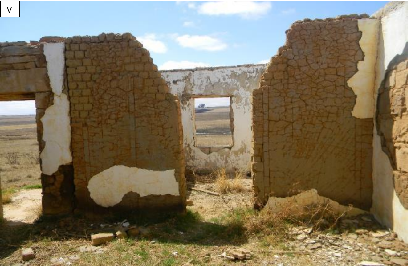
Plate 22: Photo V , showing section of the building which are structural not sound. Note that restoring the building may be difficult and expensive should the applicant wish to protect the historical building.
