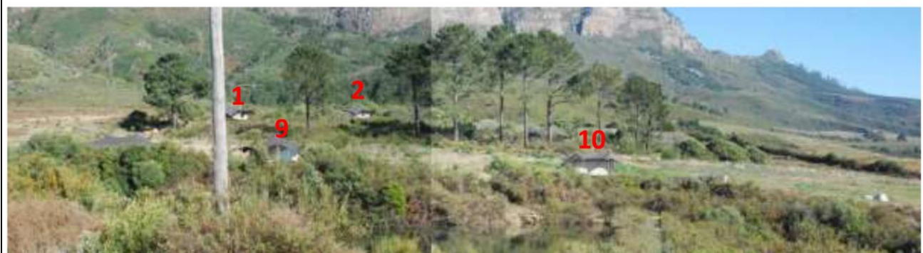
Figure 26: View from across the dam showing the visibility of Tent Structure 1, 2, 9 & 10 (source: Winter et al., 2021)
