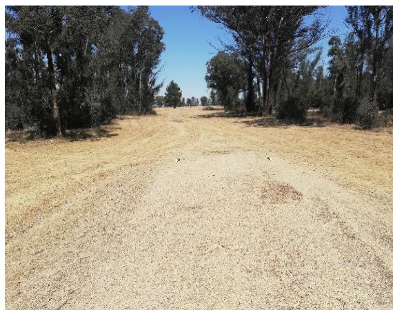
Figure 17: Road on the site.
