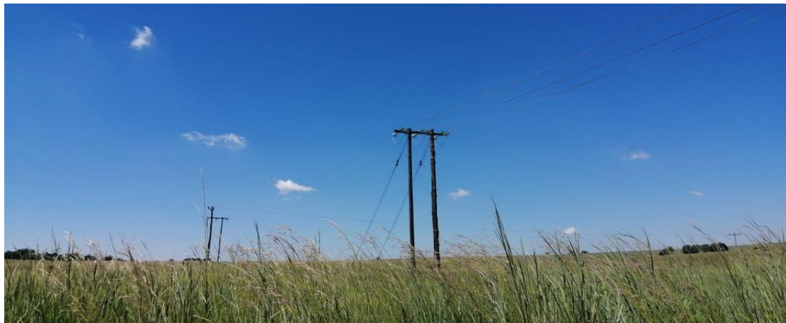
Figure 39: Infrastructures identified within the proposed project area.
