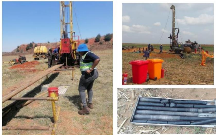
Figure 1: Example of drilling equipment and site setting (Singo Consulting (Pty) Ltd, 2023)
