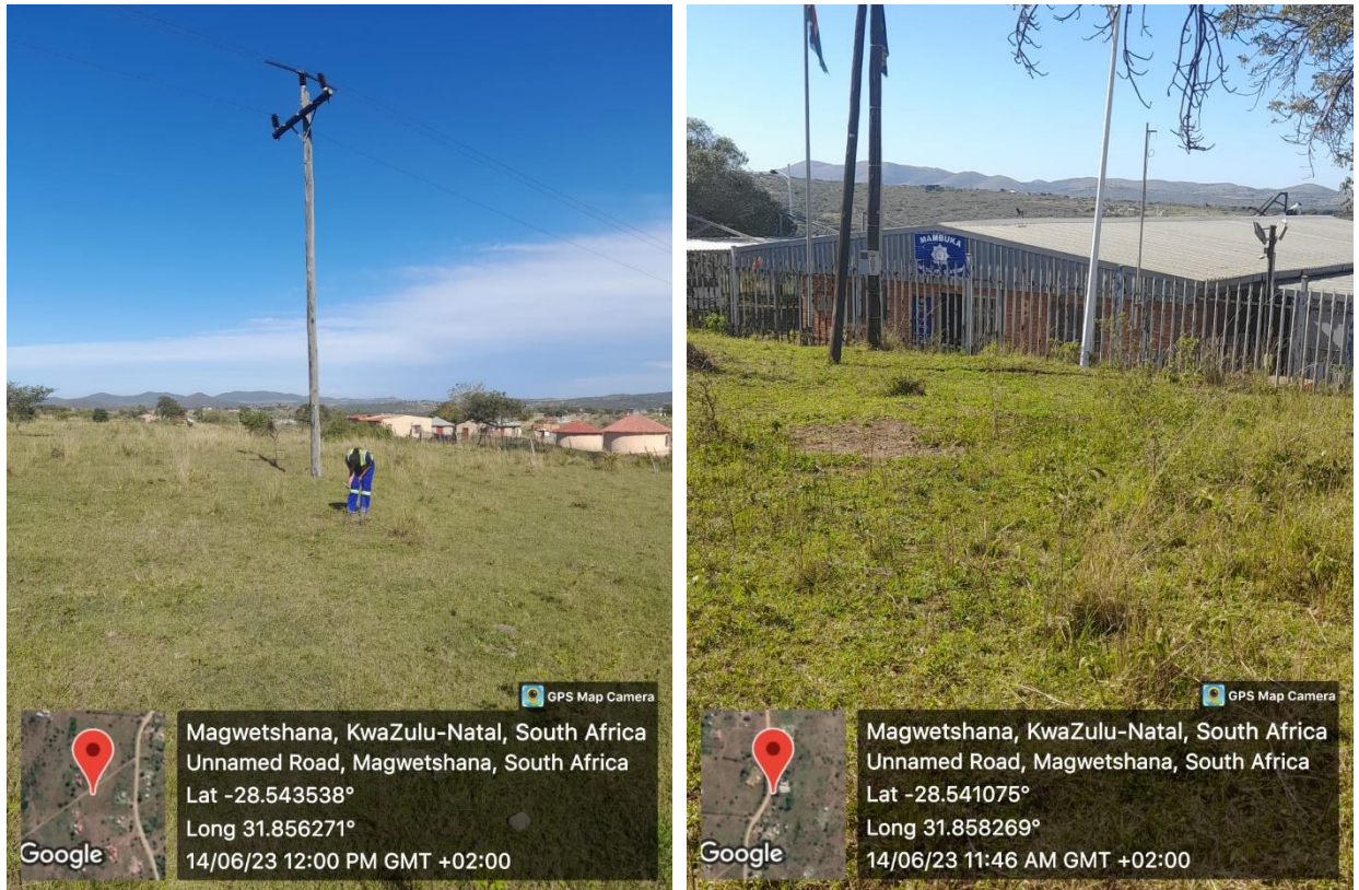
Figure 44: Infrastructures observed on site (Singo Consulting (Pty) Ltd, 2023)
