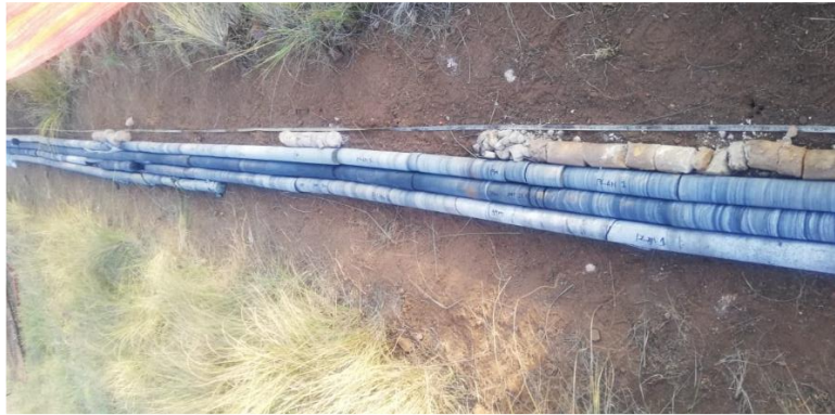
Figure 6: Typical example of borehole drilling ( Singo Drilling, 2023 )
