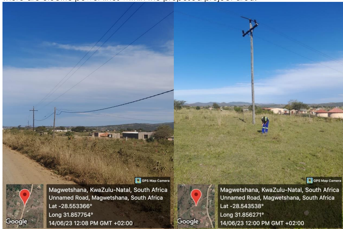
Figure 46: Powerline identified within the proposed project area (Singo Consulting (Pty) Ltd, 2023)
