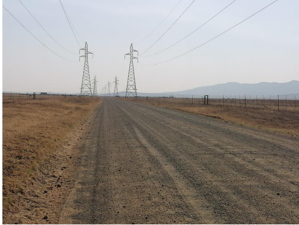
Figure 29: Types of land uses observed on site
