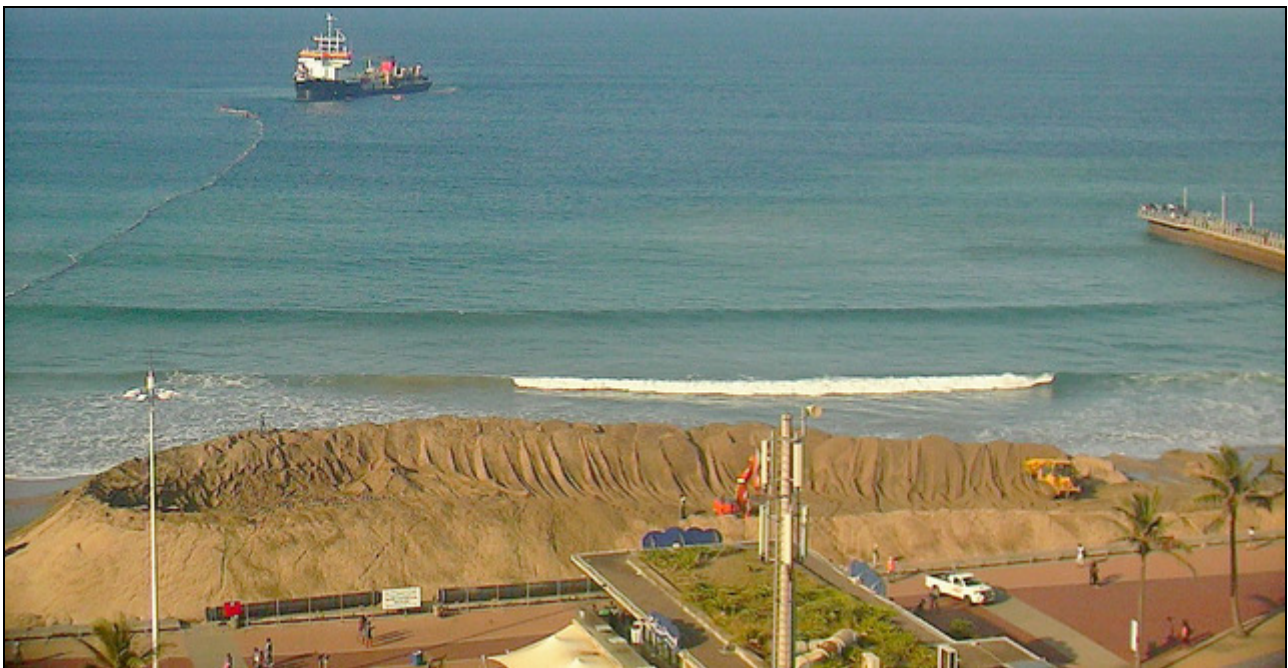
Figure 4: Emergency sand pumping directly to Durban's central beaches, May 2018 (image: swell.co.za).
