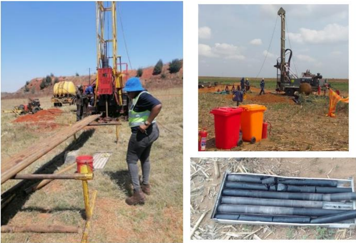
Figure 8: Example of drilling equipment and site setting (Singo Consulting (Pty) Ltd, 2022)
