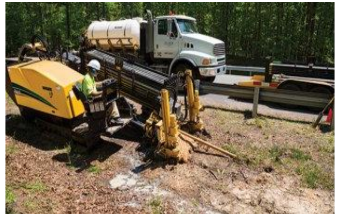
Figure 5: A typical illustration of Directional drilling.
