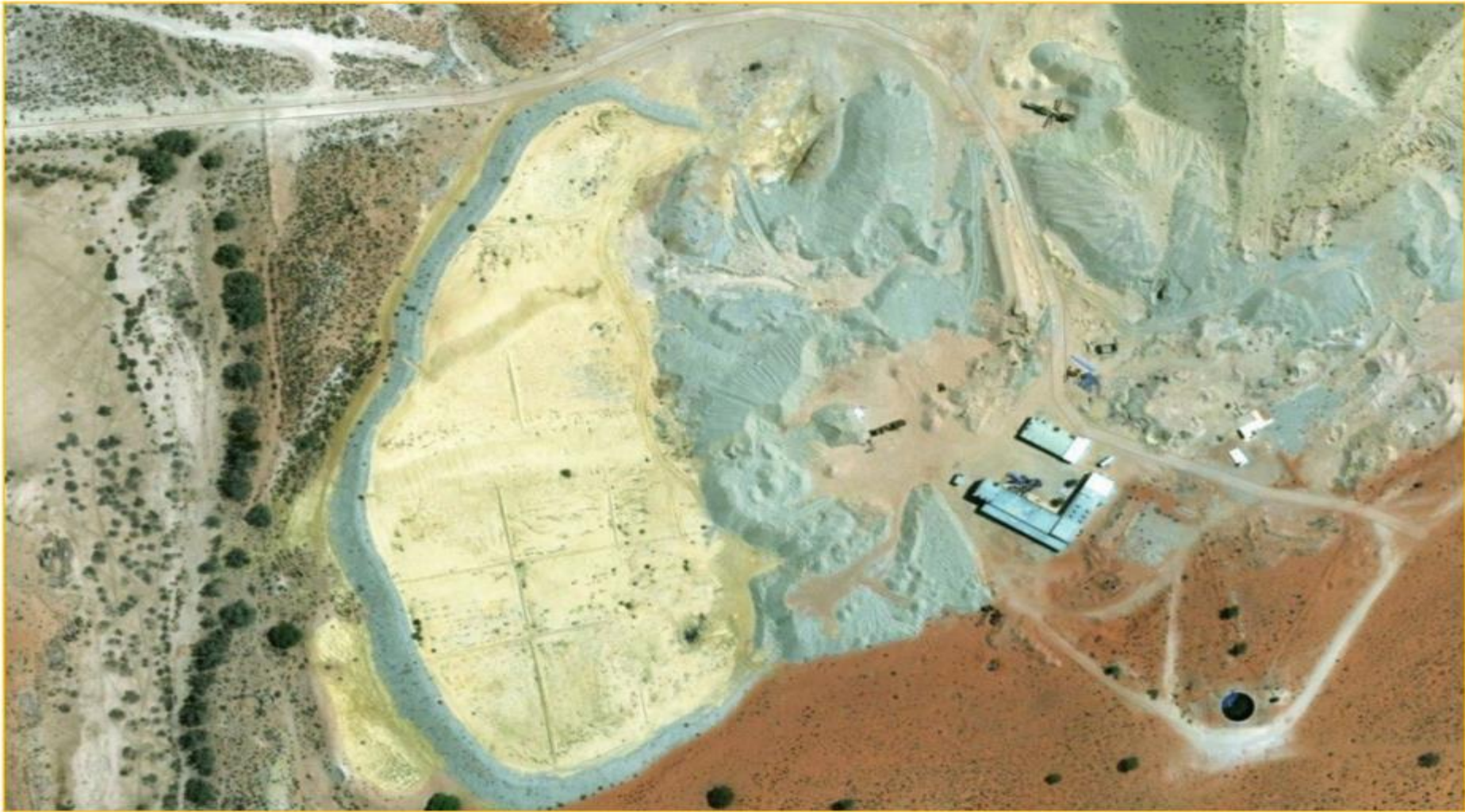
Figure 2. A plan indicating the overall location and extent of listed activities and main infrastructure Mine logistics, Security and Access Control
