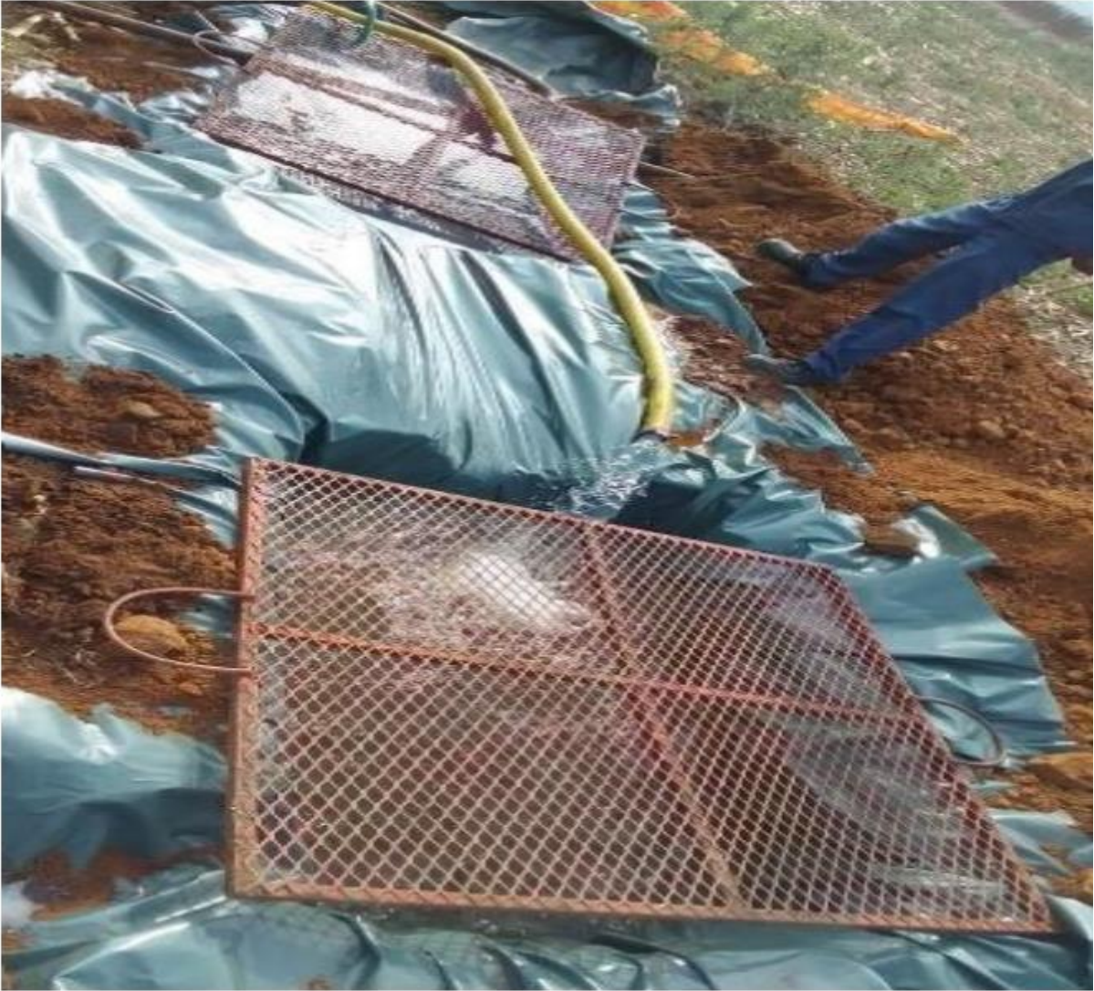
Figure 38: Sump lined with impermeable layer.
