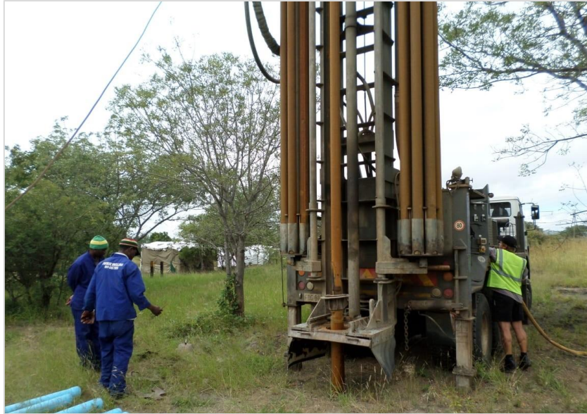
Figure 13: Example of drilling machinery
