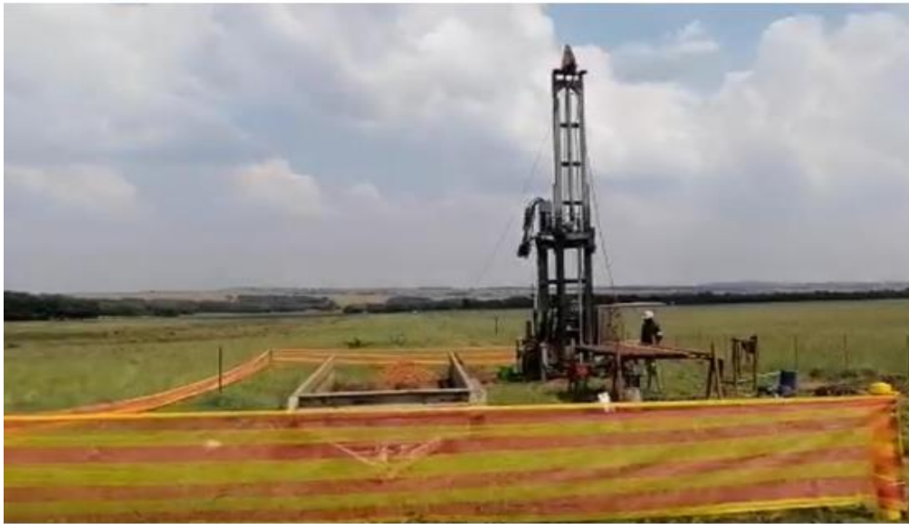
Figure 9: Example of temporary fence
