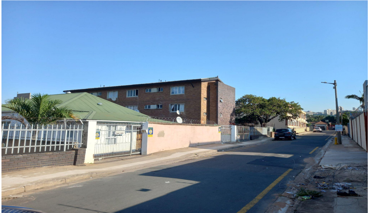
THREE STOREY BLOCK OF FLATS 3 PROPERTIES AWAY FROM OURS ON THE LEFT HAND SIDE
