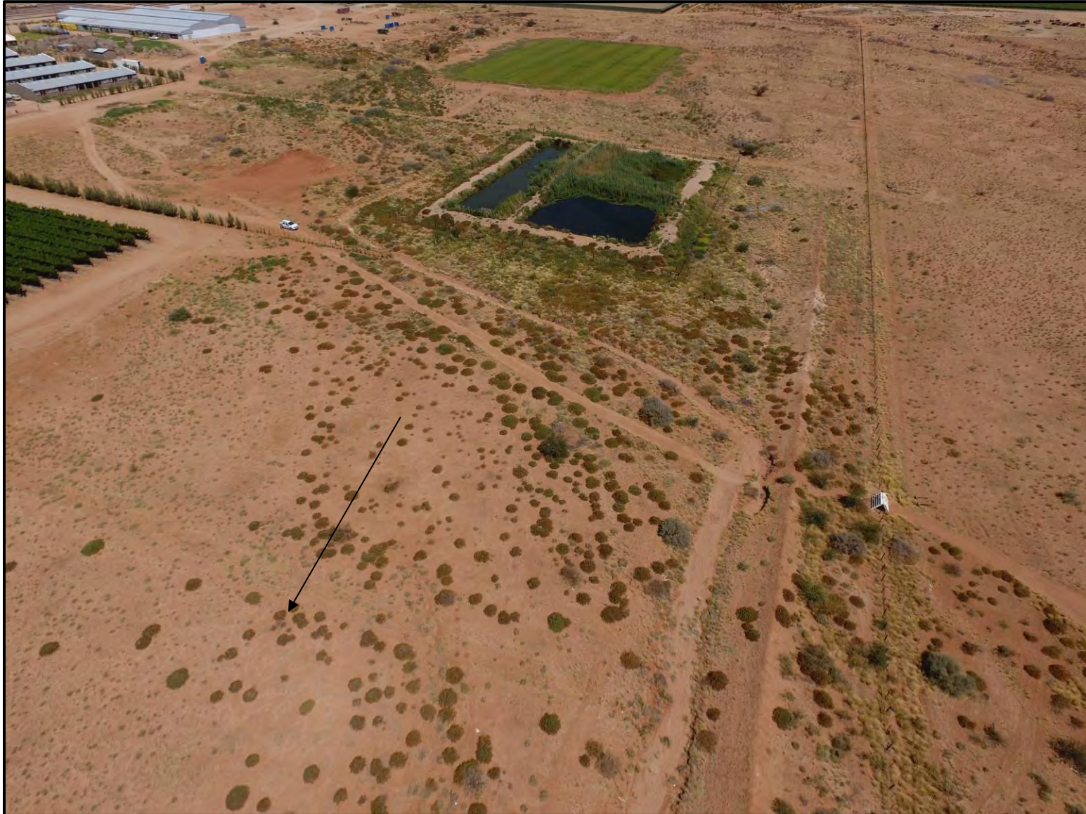
Existing evaporation pond and location of new pond (black arrow) – Drone footage
