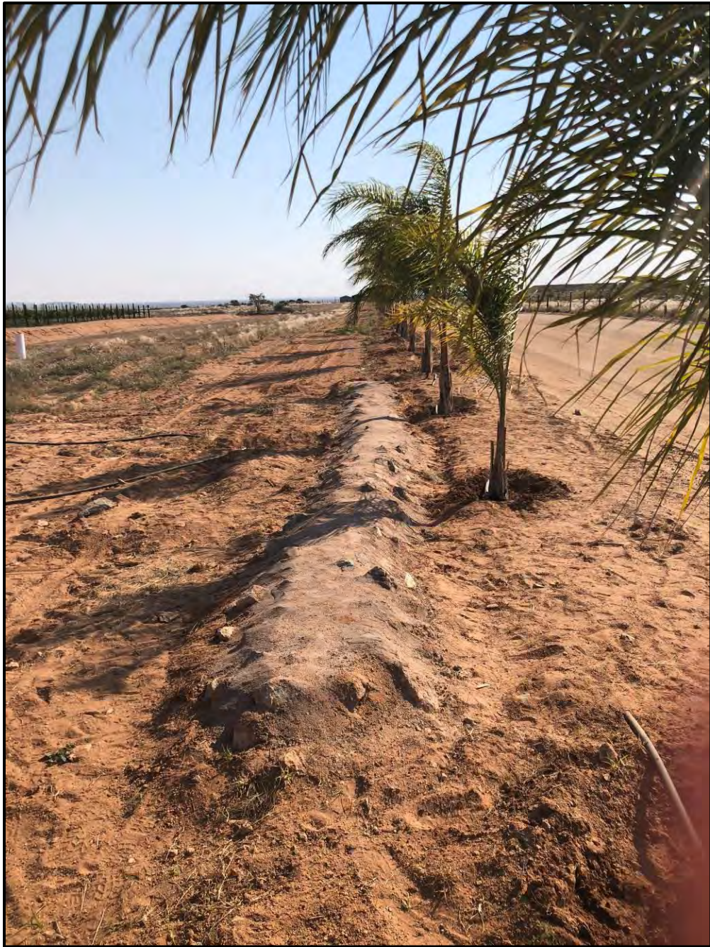
Storm water berms along the access road
