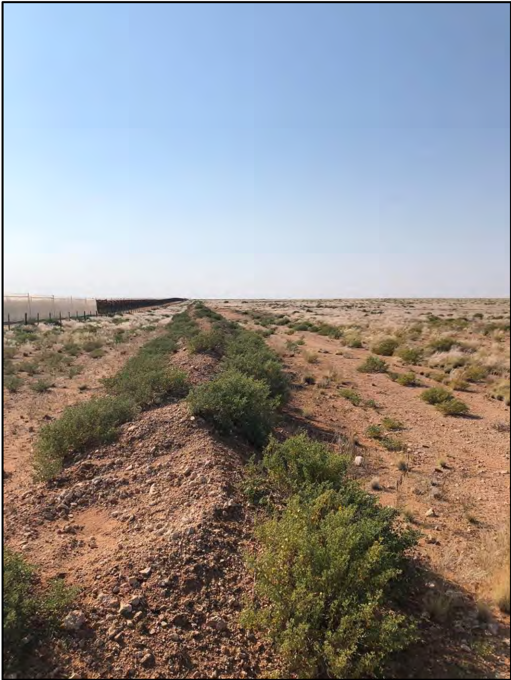
Stormwater berm at southern boundary
