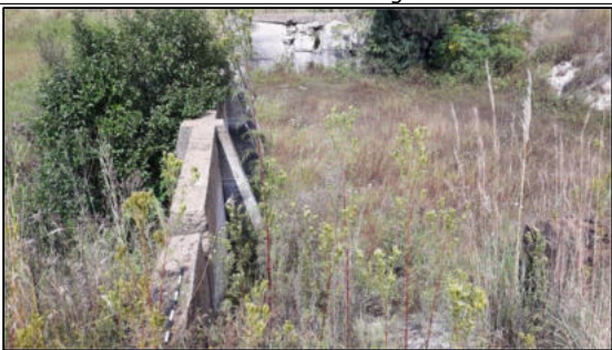
Photo 6. Remains of an old dam
