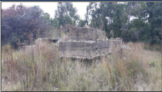
Photo 4. Remains of old mining infrastructure
