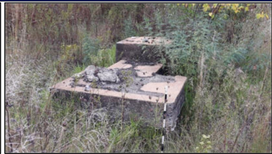
Photo 5. Remains of concrete foundation blocks
