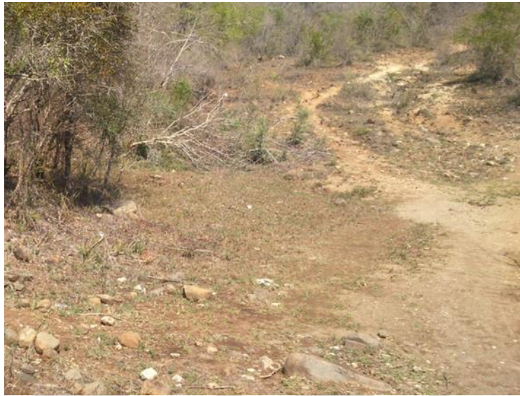
Figure 2: Image showing an exposed area where one of the proposed crossings will be constructed.
