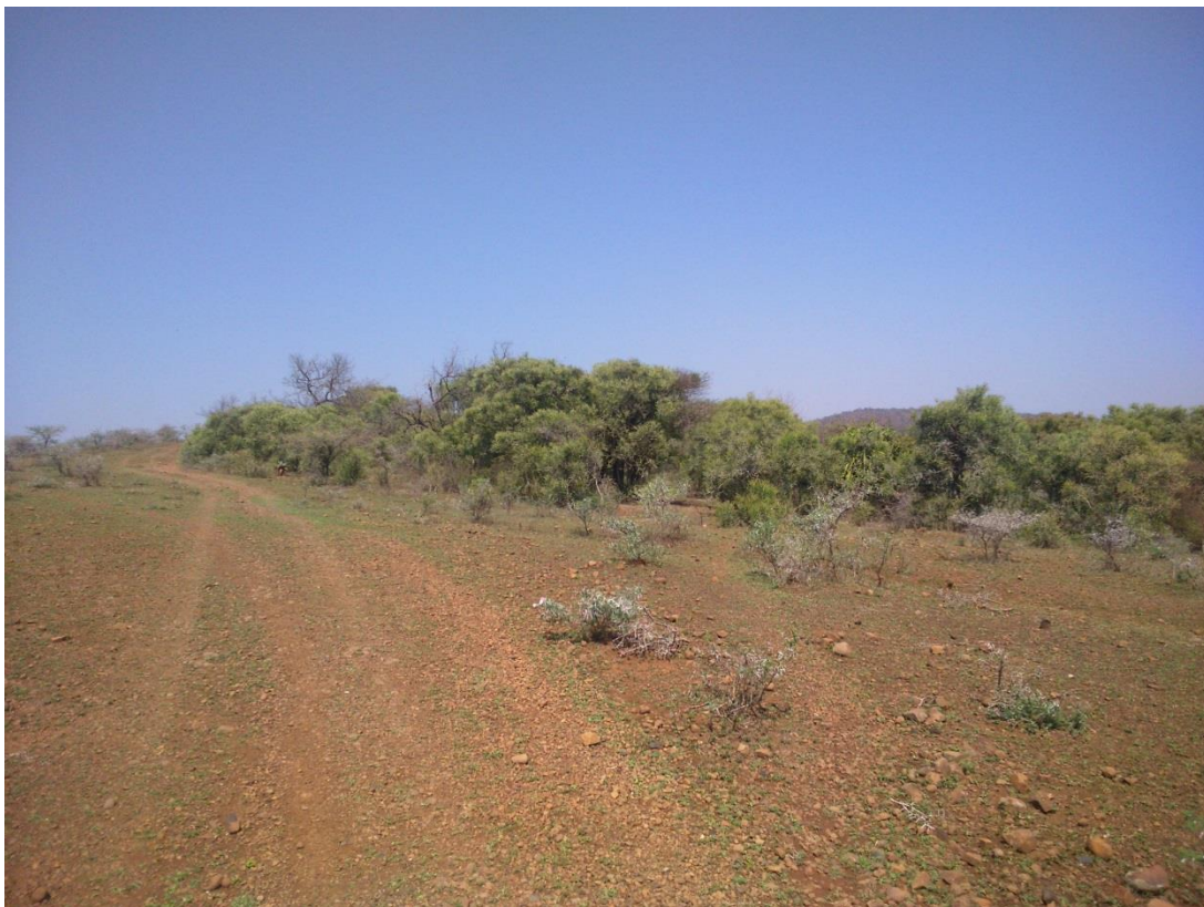
Figure 2: Image showing a stretch of the proposed road to be engineered into a formal gravel road.
