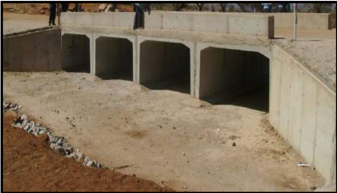
Photograph 1: showing example of a portal causeway structure.
