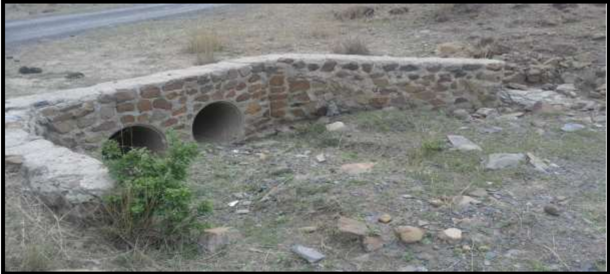
Photograph 3: Showing stone pitched pipe culverts with headwalls.
