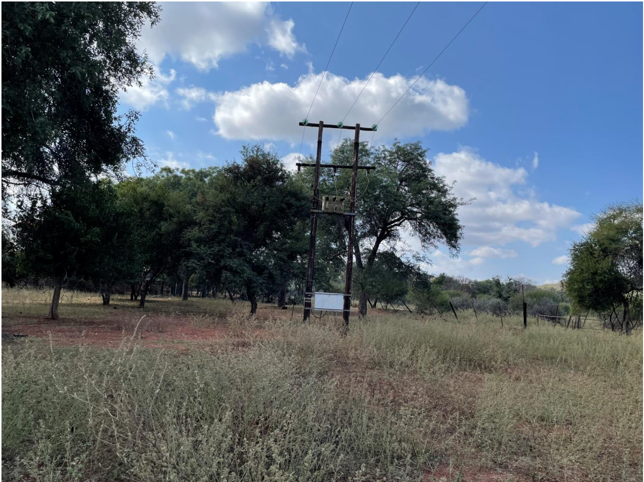
Figure 7: Existing Eskom power-lines on site
