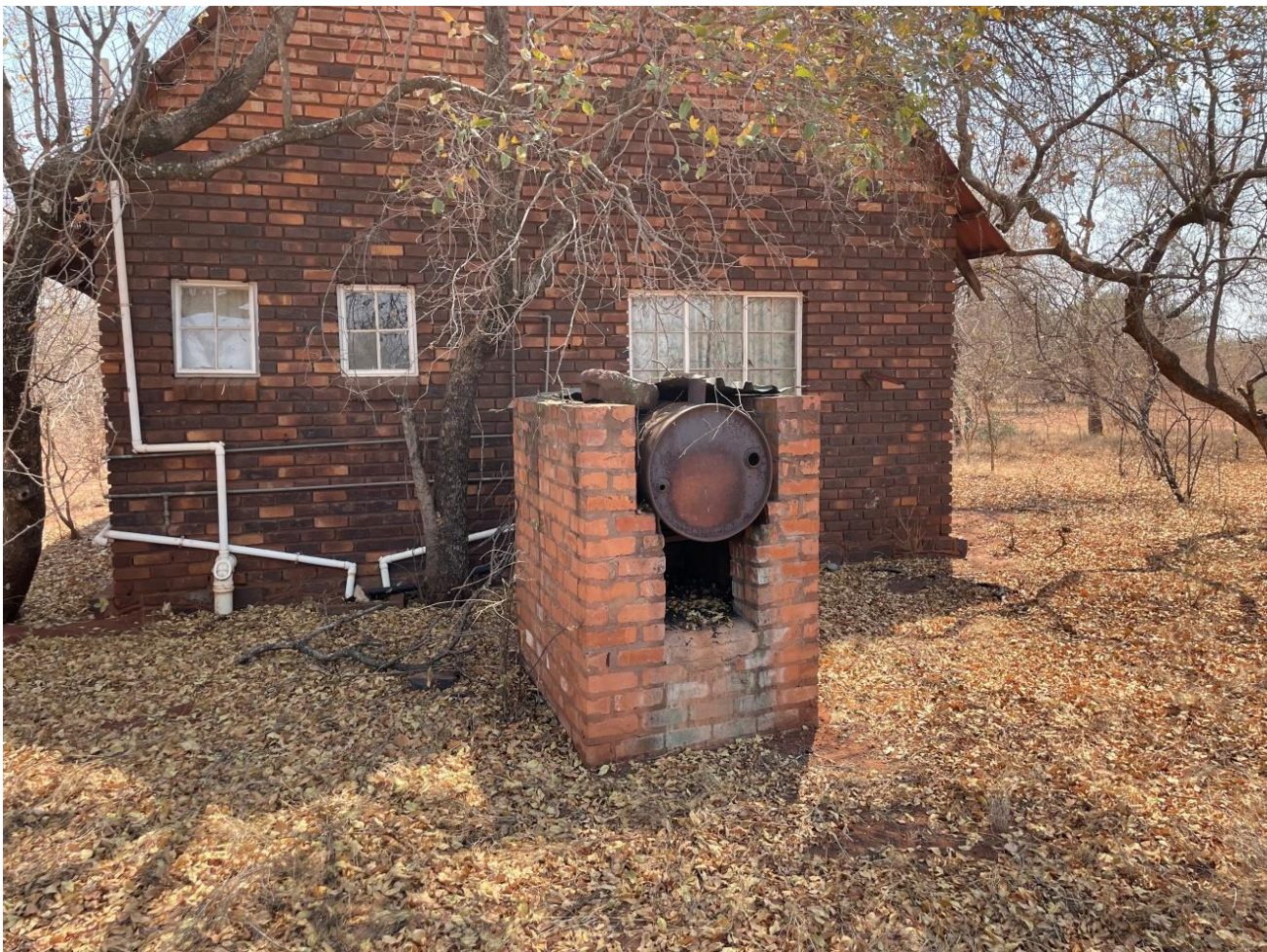
Figure 34: Current infrastructure within the applied area
