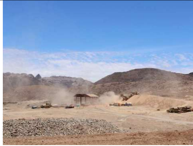
Photo 8: Overview of processing plant including ramp and associated infrastructure at Section 1.
