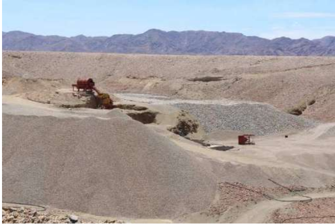
Photo 17: Old Section 2 processing plant
