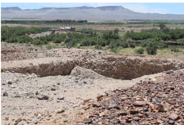
Photo 15: Mined trench being backfilled before spreading topsoil
