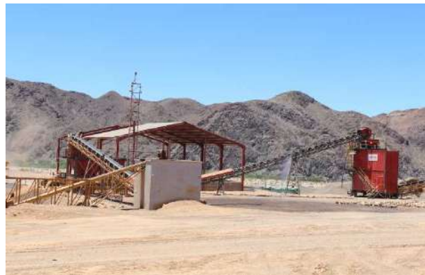
Photo10: Processing Plant (Final Recovery Plant) and steel structure with water spraying to allay dust.
