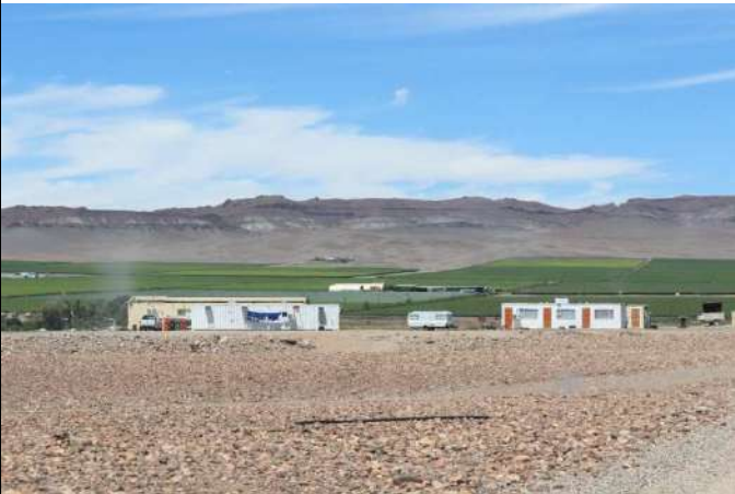
Photo 3: Containerized accommodation units
