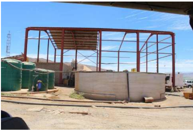
Photo 11: Steel structure, x 4 JoJo Tanks and 150m 3 steel dam
