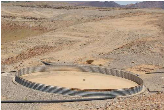
Photo 19: Steel dam (old)
