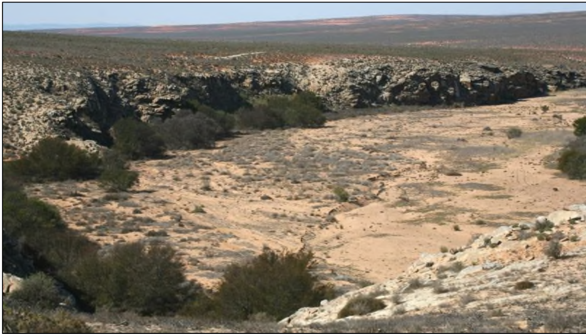
Figure 11. Looking across the Buffels River just to the south of the grid connection corridor crossing point, near the existing Gromis substation. The double-circuit power line will be able to cross the river without impact to the bed or rocky sides.
