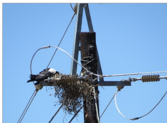
Photo 1-2: Example of dangerous power line configurations that should be avoided on any low-voltage overhead lines. A Pale Chanting Goshawk (right) perch-hunts inside a live loop – while a Pied Crow (right) lies electrocuted below a similar live loop.
