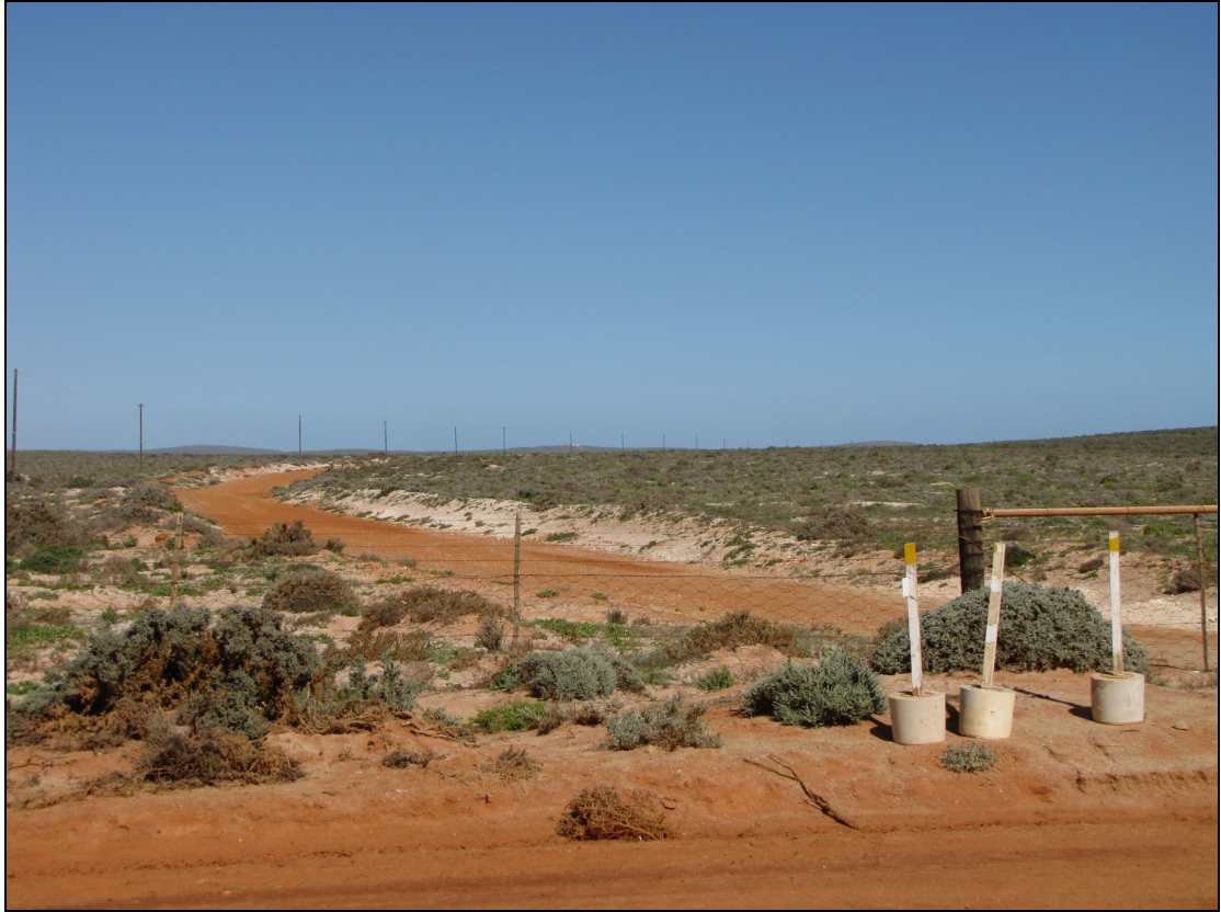
Figure 2: The general environment and existing power lines in close proximity to the 300m corridor.
