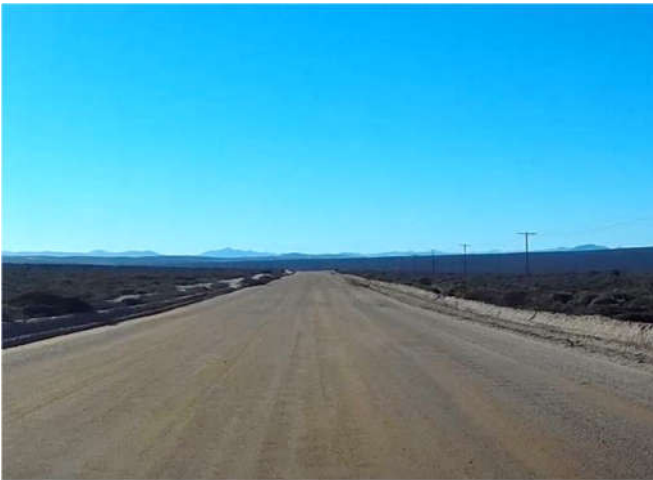
Photograph 2-11: MR751 Gravel Section
