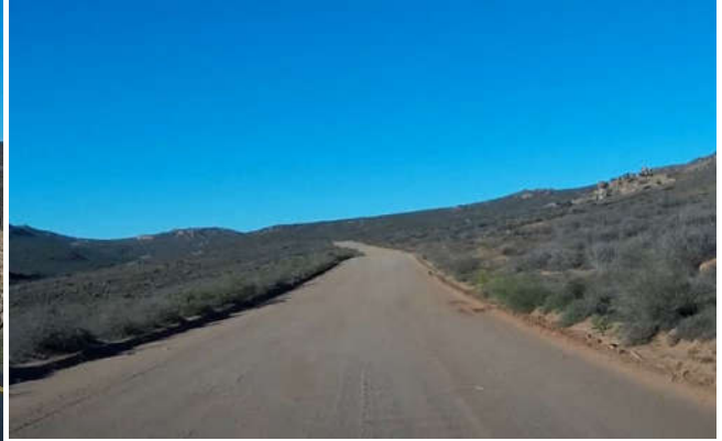
Photograph 2-10: MR739 Gravel section
