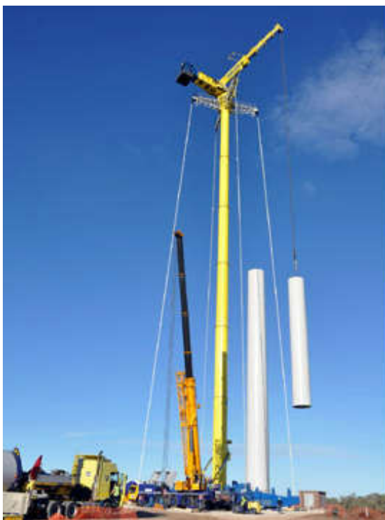
Figure 3-6: Cranes at work (Source: Author's photograph)
