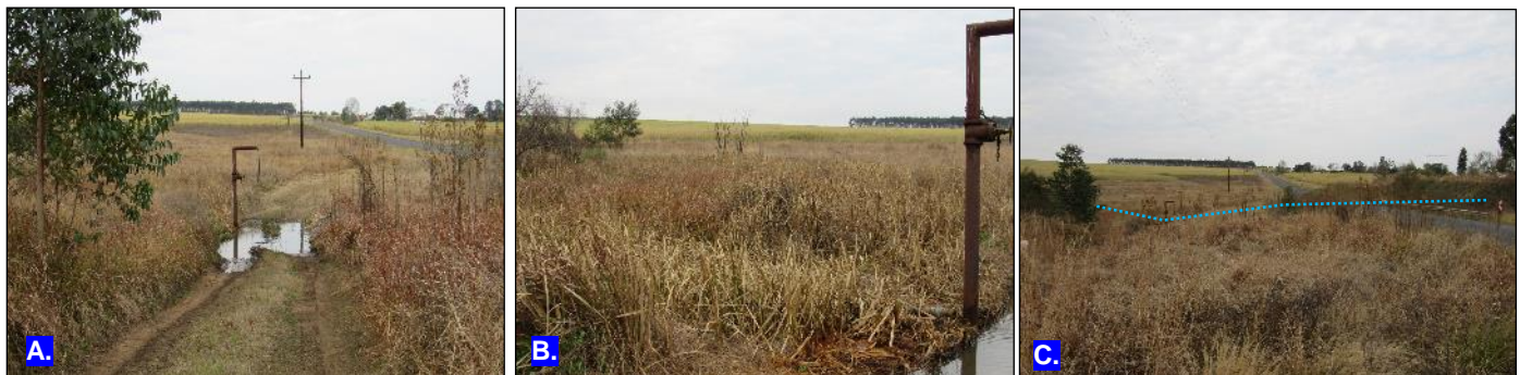
(a): Overview of WC2 adjacent to the P154 (b): Upstream of WC2 where the watercourse opens out into a valley-bottom wetland (c): Blue dotted line showing the location of the watercourse as it flows underneath the P154 towards the main Mhlalane River.
