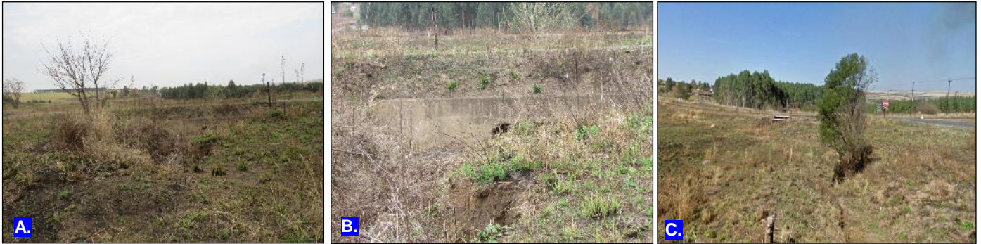
(a): Non-perennial drainage line crossed at WC3 (b): Existing pipe underneath the P154 at WC3 (c): Downstream view at WC3 looking towards Schroeders Road.
