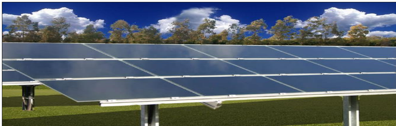
Figure 6 Frontal view of PV arrays mounted on fixed mounting systems
