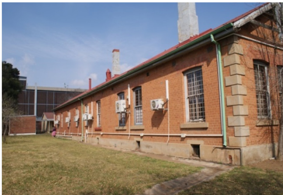
Image 6: Main Building Family Court
