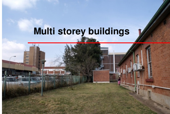
Image 17: Image illustrating the height of surrounding buildings
