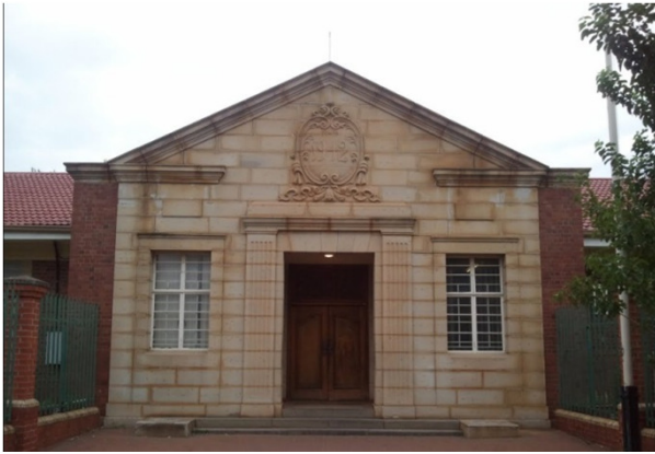
Image 10: Entrance to existing Magistrates Court
