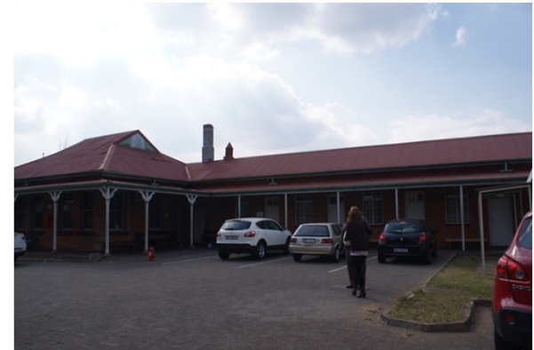
Image 4: Family Court to be restored (old Police Station)
