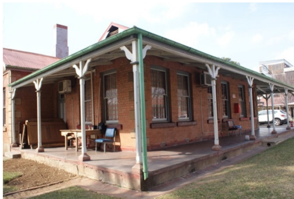
Image 3: Elevation of the stoep area
