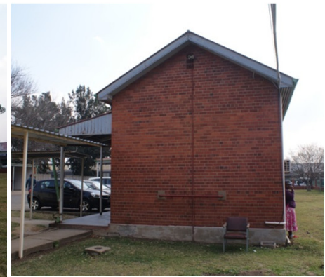
Image 9: North Eastern view – back of building
