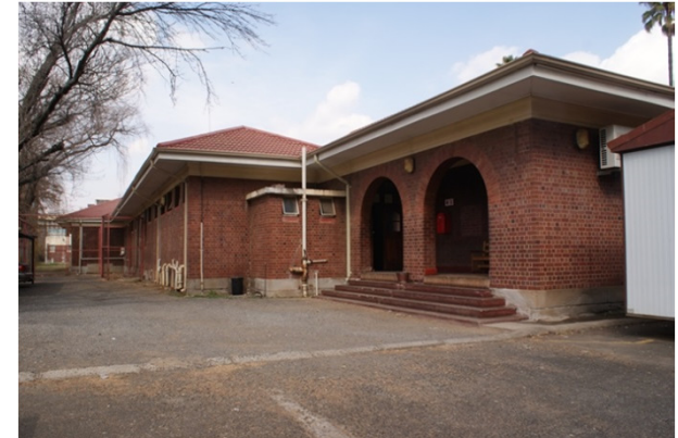
Image 15: Northern view of addition (to be demolished)
