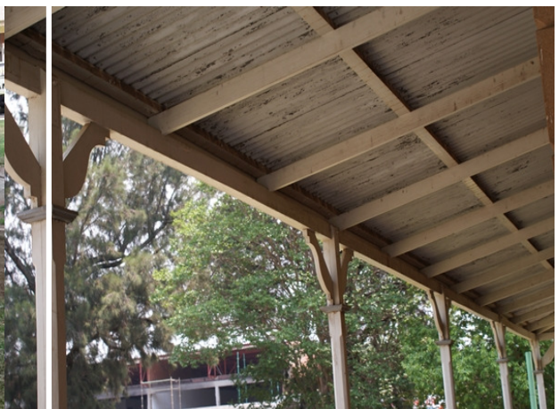
Image 15: 9-Timber beams & purlins
