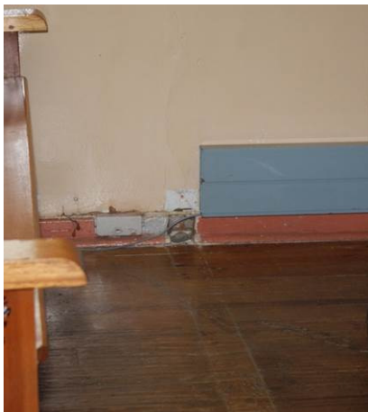
Image 4: Damaged skirting
