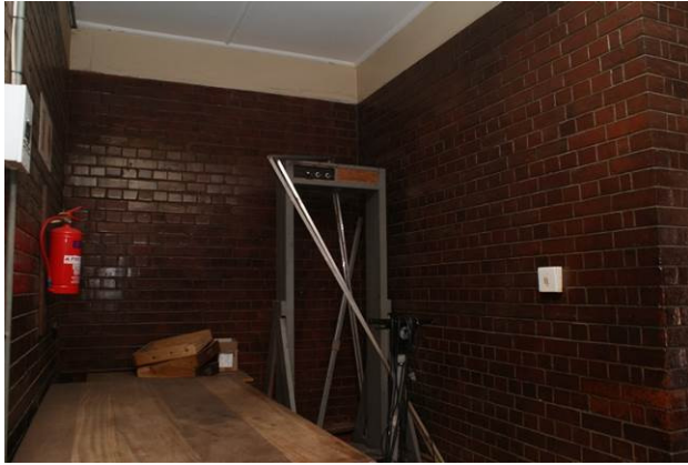
Image 31: Entrance to be reopened(interior)
