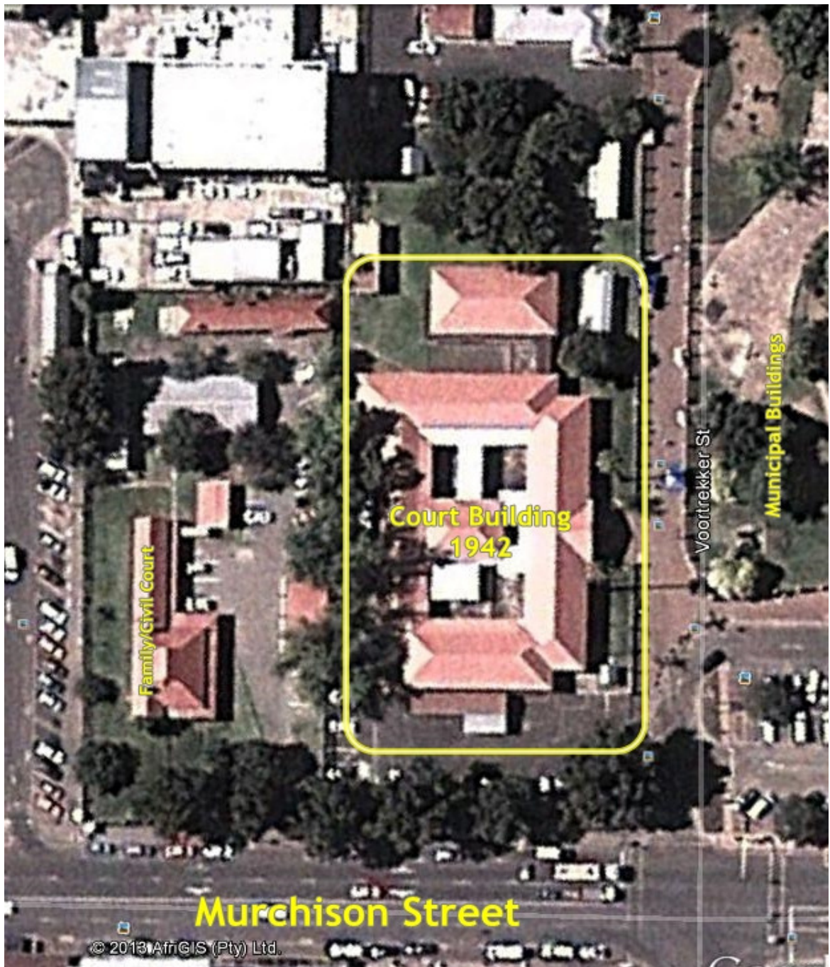
Image 38: Location of the building
