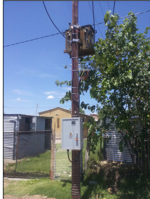
Figure 4: Existing transformer
