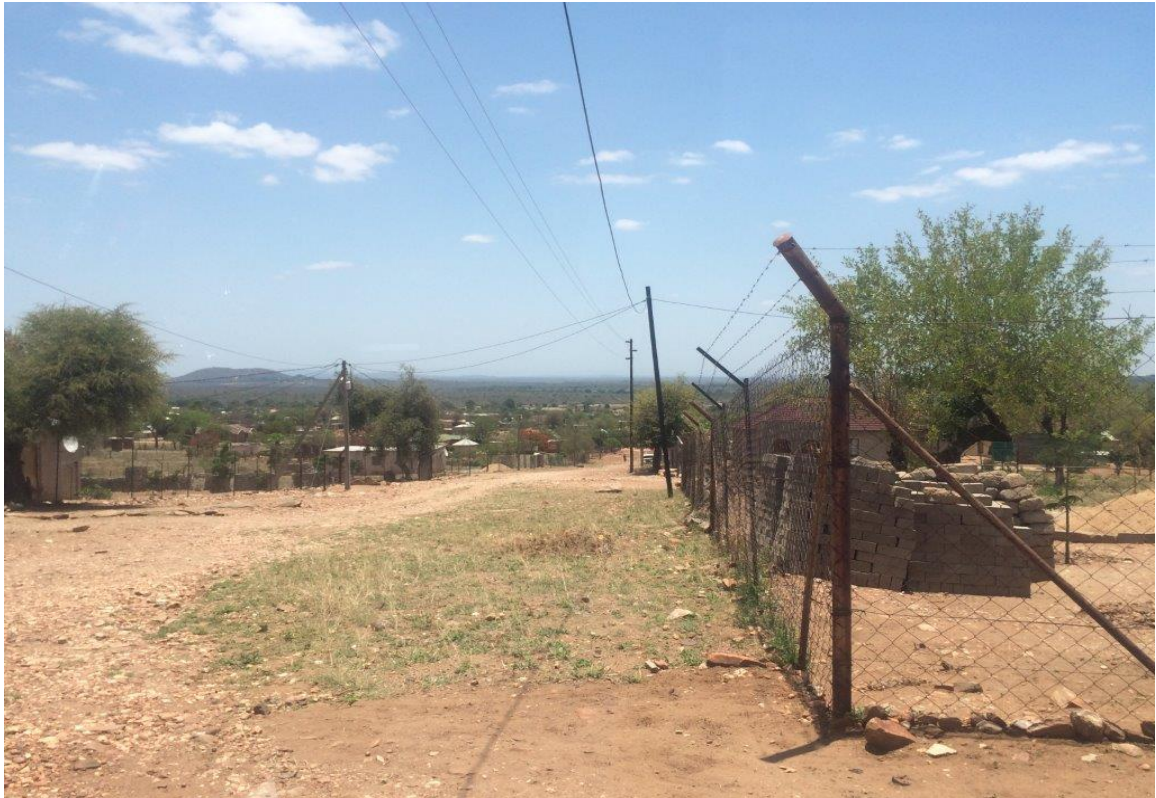
Picture 1: Shows the existing MV and LV lines as well as the access road on site
