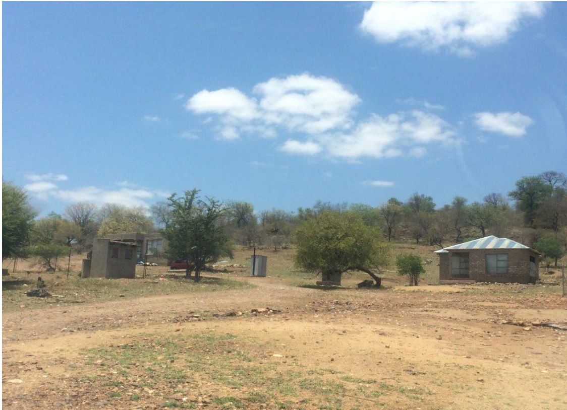
Picture 5: Houses to be electrified on site
