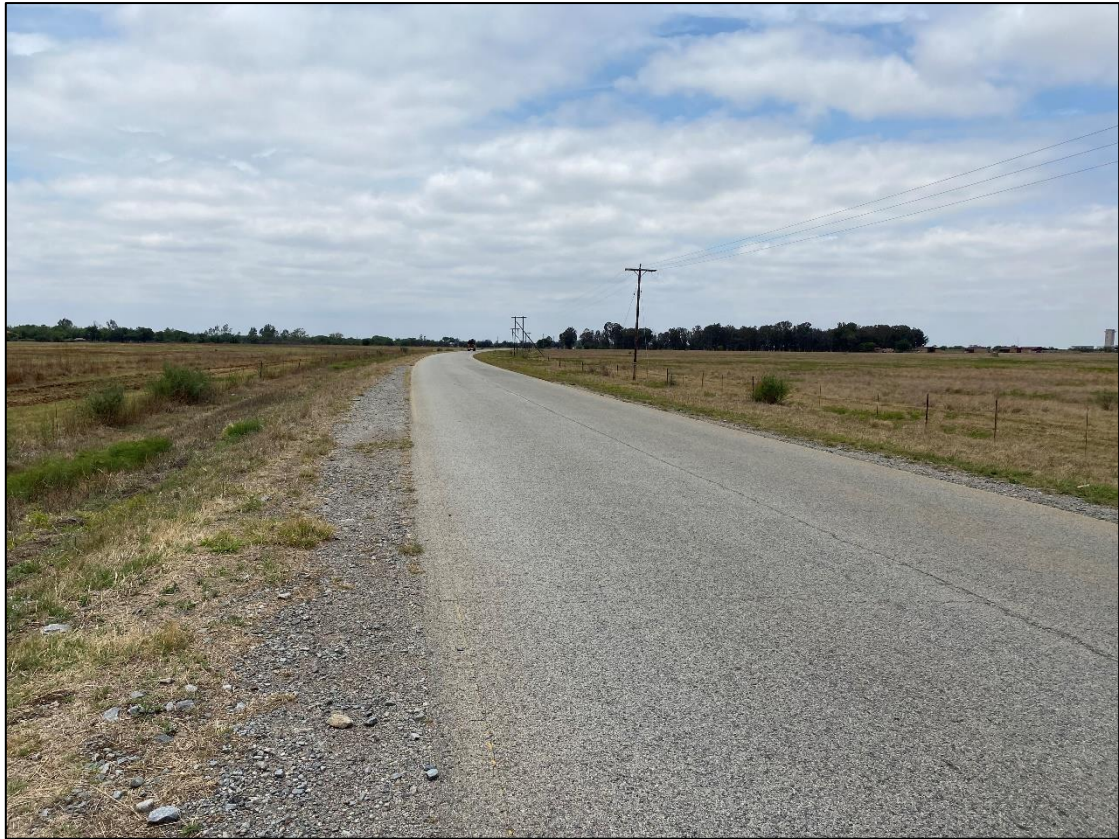
Plate 2: Stokkiesdraai road access route taken towards the north-east.
