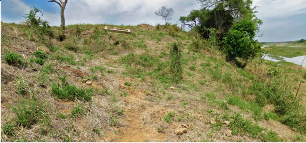
Overgrazed and trampled macro-channel
