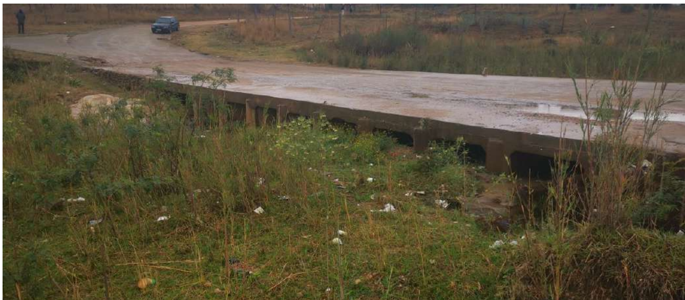
Figure 10 Stream 1, culvert 4, barrels 9No. 1200mm high x 1200mm wide
