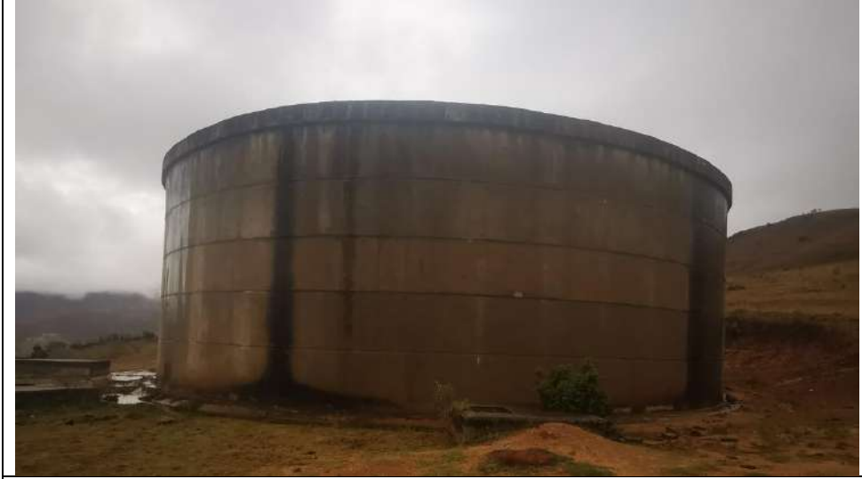
1.5Mℓ reservoir, Ward 16 Nhlazatshe, Mpumalanga
