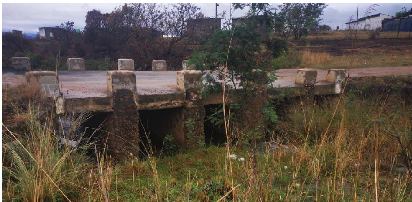
Figure 8 Stream 1, culvert 3, barrels 5 No. 1200mm high x 1200mm wide
