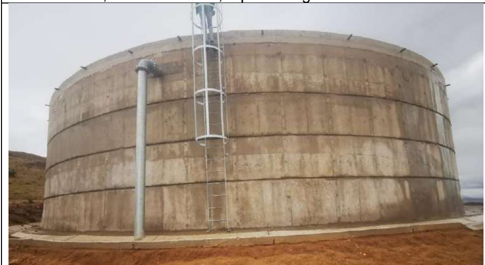
2Mℓ reservoir, Ward 16, Nhlazatshe, Mpumalanga.
