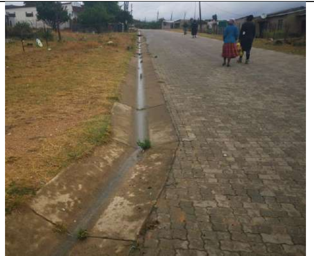
Typical block paving road, Nhlazatshe
