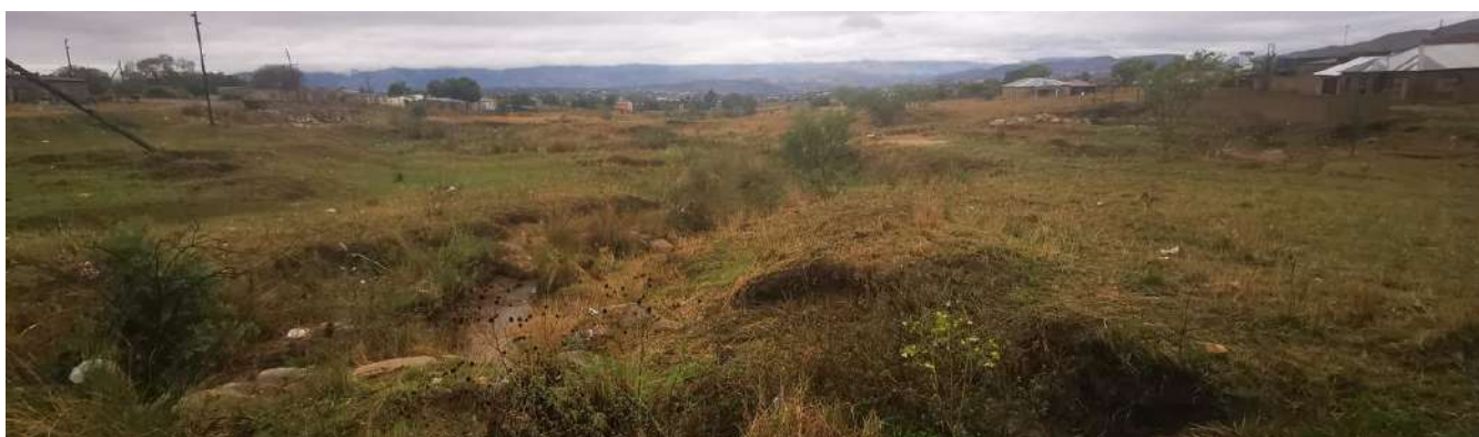
Figure 7 Stream 2, downstream of culvert 2
