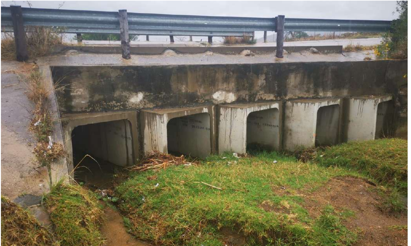
Figure 4 Stream 3, culvert 1, barrels 5No. 1200mm high x 1200mm wide
