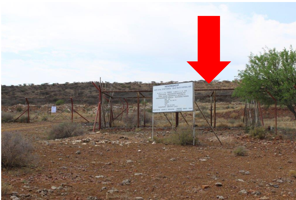
Plate 1.1: The access gate leading to Niekerskshoop landfill, the landfill is in the background, site is fenced off. Arrow shows an equipment storage area
