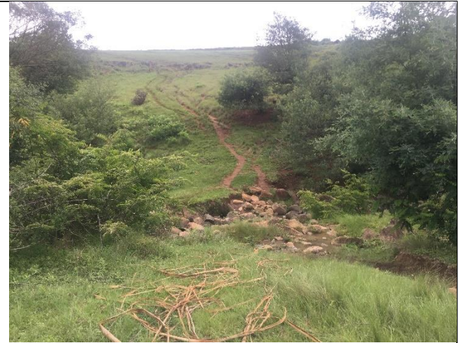
Plate 2. Image looking north overlooking the Proposed road alignment at the uMvubukazi River watercourse crossing towards the mid-point of the road construction.
