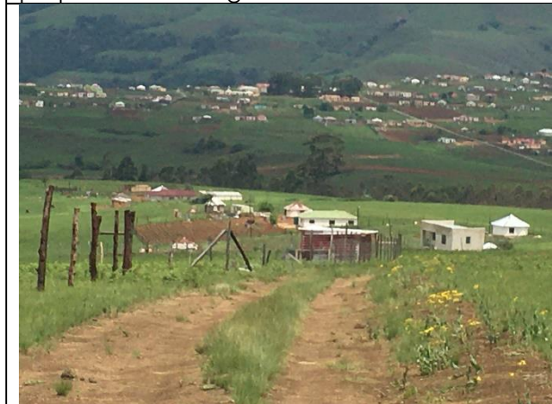
Plate 3. Image showing rural community who will be serviced by the new Nigel Access Road.
