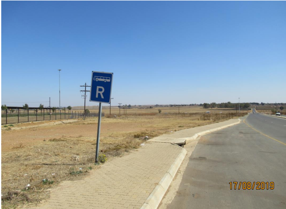
Figure 14: End point in the north (710) S26 21.190, E28 27.556
