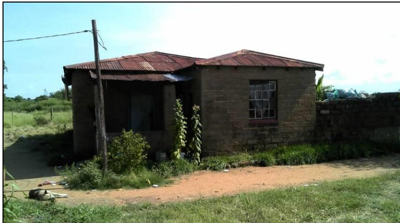
Figure 10: View of the south face of the main house on the site.
