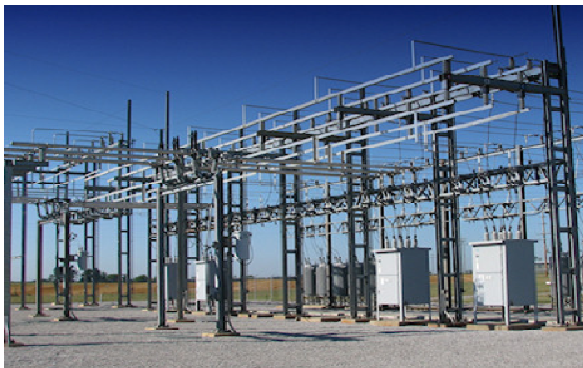
Figure 4: Illustration of a 132kV Distribution Substation
