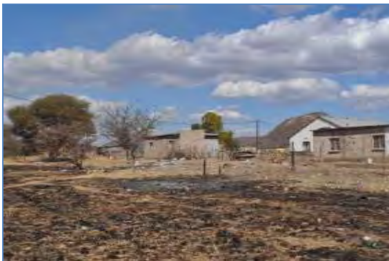
Figure 35: Poor quality buildings east of the development site
