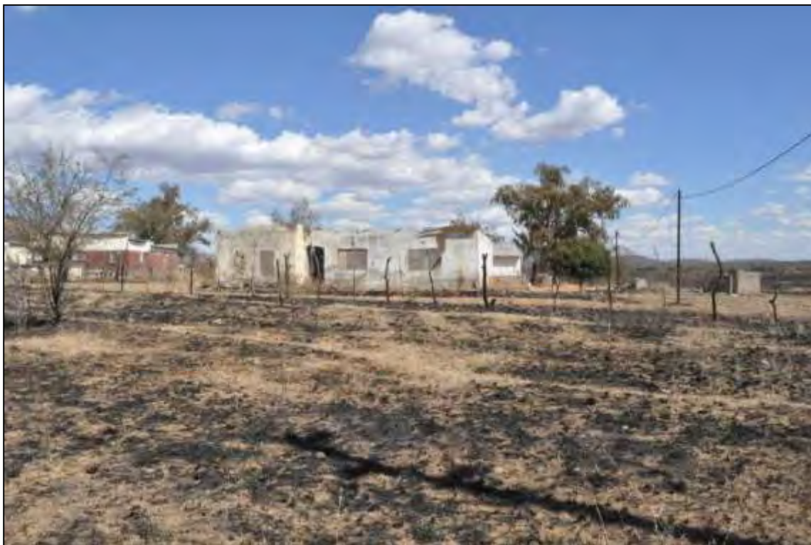
Figure 7: Derelict buildings close to the development site and transformed vegetation
