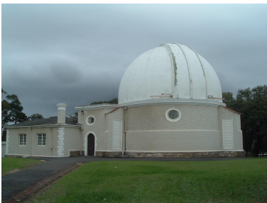
PHOTOGRAPH 1: ELEVATION OF THE BUILDING
